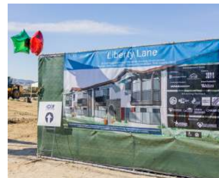
Liberty Lane Groundbreaking
